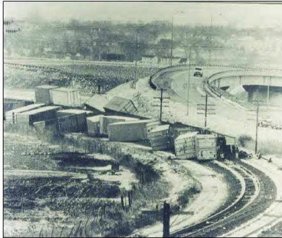
Wasatch Front, April 4-6, 1983 – 70 mph “East Winds” derailed this train in the Lagoon area. Peak gusts were recorded at 104 mph.
